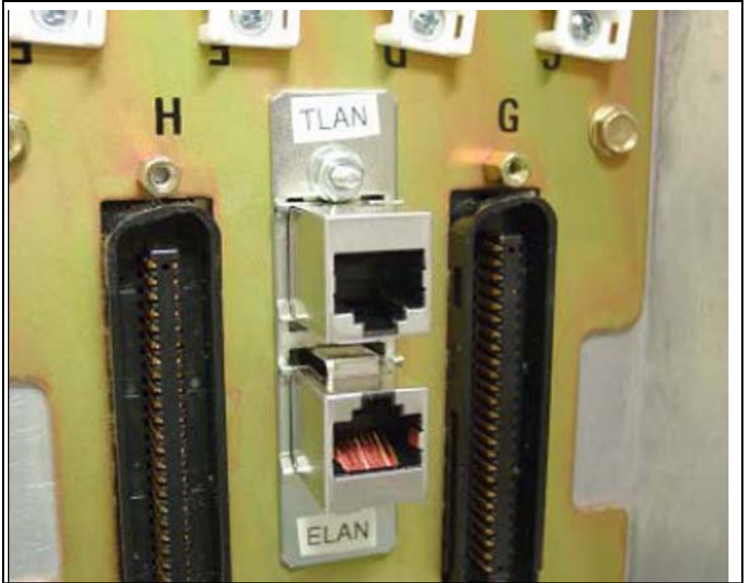
Figure 50 Installed Ethernet port adapter plate
